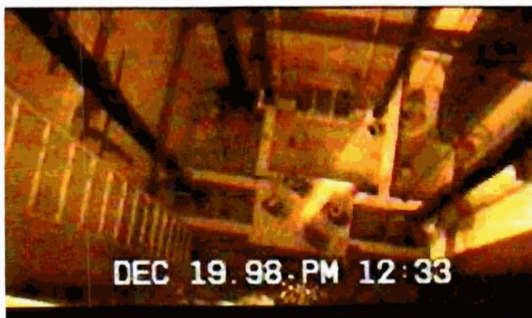
Top down view of a flooded elevator shaft and top of elevator.
